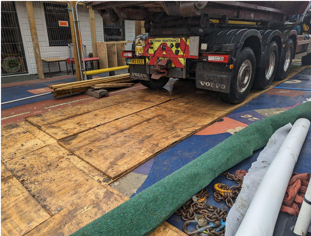
Photo 03 - Protection laid to rubberbound surface adjacent to Nursery.
