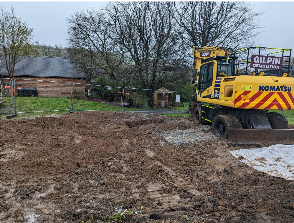
Photo 06 - Devon Lady Unit Nr2 demolished and material arisings carted from site.
