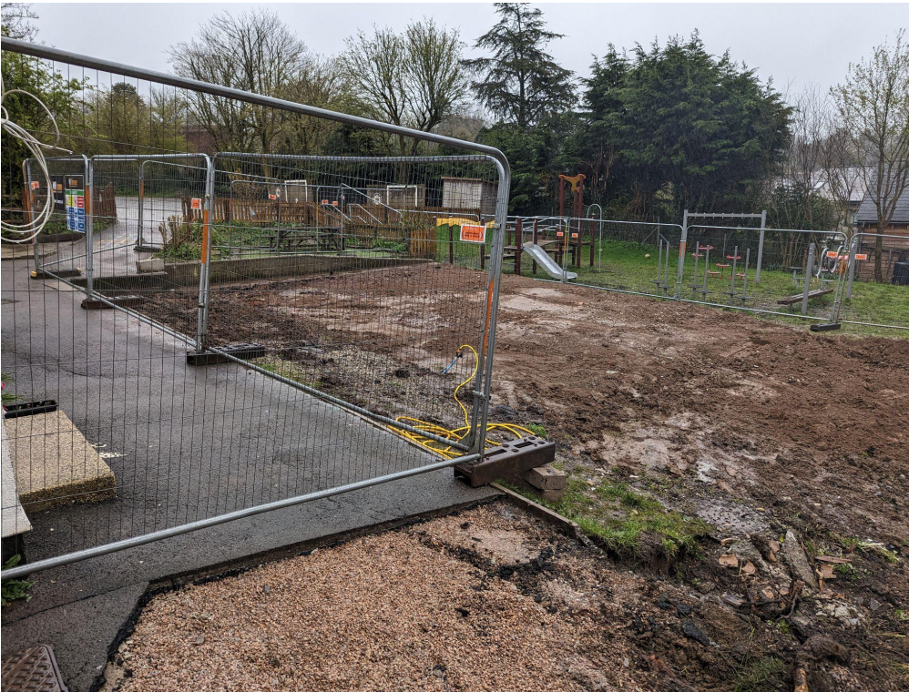
Photo 05 - Devon Lady Unit Nr1 demolished and material arisings carted from site.
