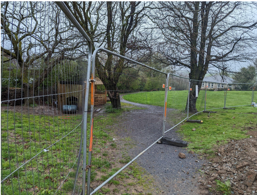
Photo 04 - Tree protection measures.
